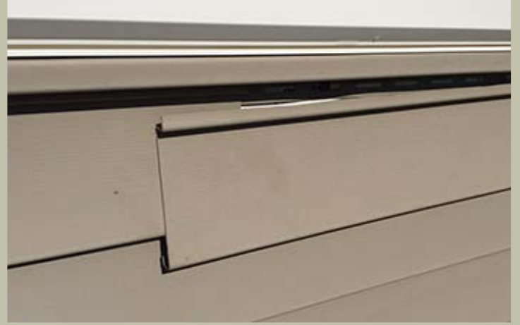
Uneven and shifting boards
