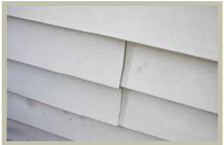
Obvious seams and gaps between planks
